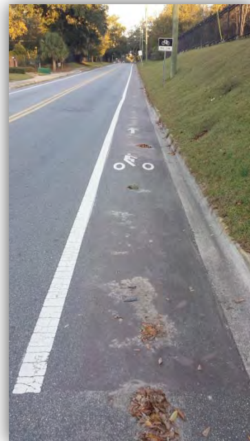
Illustration 1.24: Example of Once-Painted Bike Lane on W. Call Street. Photo Credit: Studio Team.
