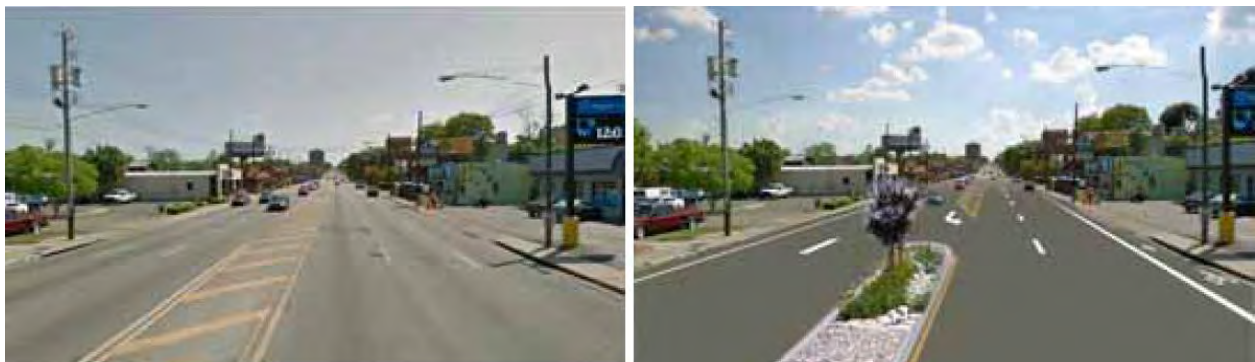
Illustration 1.40: Potential Midblock Crossings. Photo Credit: Road safety assessment 2012. Florida Department of Transportation, (2012). Road safety assessment report Tennessee Street US 90/SR 10(Ocala Road to Monroe Street).
