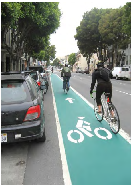
Illustration 1.33: Example of a Well-Painted Bike Lane
