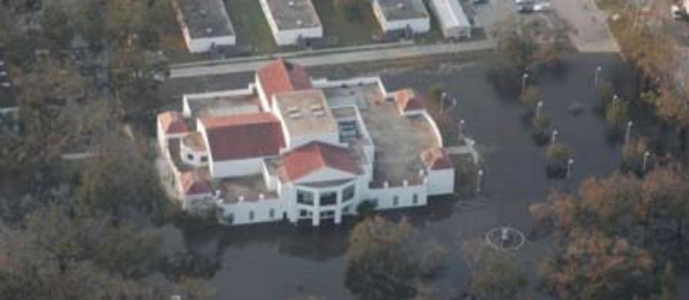
Aerial view of a flooded Dillard University days after Hurricane Katrina hit August 29, 2005.
